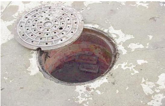
Figure 2B. Existing manhole with crumbling brick.
