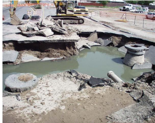
Figure 5A. Sanitary sewer backup can result in a sinkhole. These cause the most monetary damage because roads and utilities need to be replaced.
