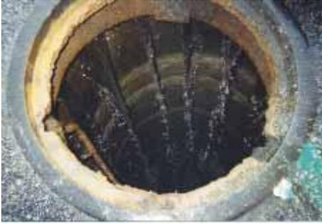
Figure 1. A manhole in very poor condition with a very high infiltration rate with cracks in the walls. This manhole would have been given a rank of “one” for condition due to the size of the cracks and a “five” for infiltration rate based on the amount of water potentially entering the structure. This structure would have been scheduled for replacement as soon as possible.
