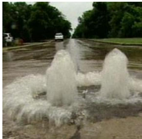
Figure 5B. The manhole is overflowing and flooding because of a system that was over capacity.
