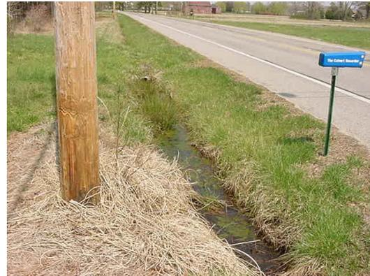
Figure 3. Here ditches are used for drainage along roadways.
