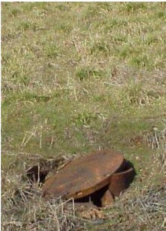
Figure 2A. Existing manhole with a broken lid and insufficient casting.
