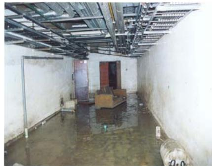
Figure 3. Flooded basement.
