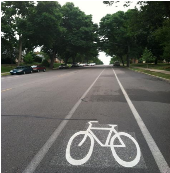
Figure 5. A typical bicycle lane in the City of Minneapolis will be clearly marked by a pavement symbol illustrated above. These lanes are commonly flowing in the same direction as traffic.
