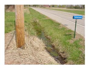
Figure 3. Here ditches are used for drainage along roadways.
