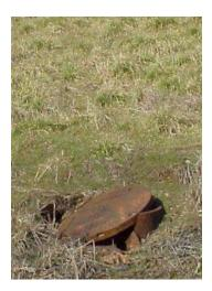
Figure 2A. Existing manhole with a broken lid and insufficient casting.
