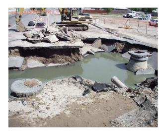
Figure 5A. Sanitary sewer backup can result in a sinkhole. These cause the most monetary damage because roads and utilities need to be replaced.
