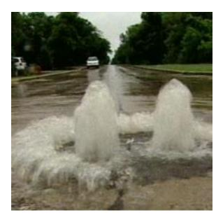
Figure 5B. The manhole is overflowing and flooding because of a system that was over capacity.
