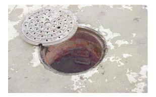
Figure 2B. Existing manhole with crumbling brick.
