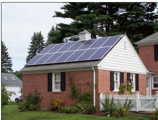
Figure 5. Sample residential rooftop PV system. Image provided by Gerdes (2012).
