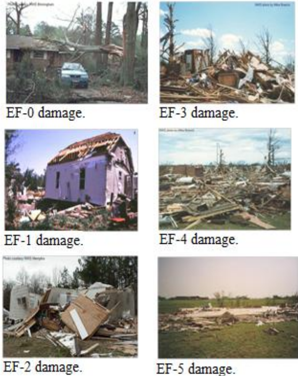
Figure 1. The figure illustrates the Enhanced Fujita Scale with an example of damage (Weather Underground, 2012).
